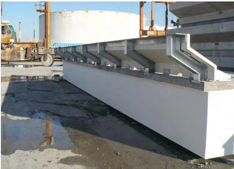
the weight of a conventional 30-foot prestressed concrete span. BNSF wants to handle the longer span with its existing on-track cranes. The designers noted that in the previous span, approximately one-third of the concrete was in the arch, one-third was in the deck and one-third was in the ballast curb. The ballast curb became an obvious target for weight reduction.
