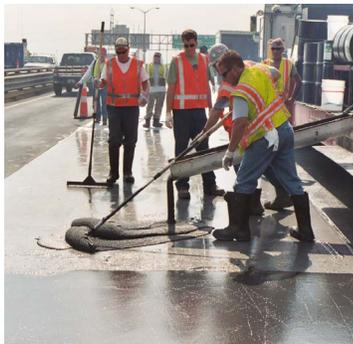
T-48 is comprised of a blended filler powder that forms a slurry when mixed with the polymer resin and broadcast with a coarse-wearing aggregate.
