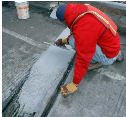
Partial or full depth applications can be accomplished in a single pour restoring the integrity of deteriorated PCC structures.
