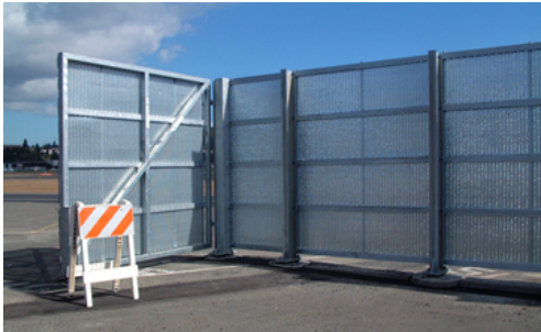
The Double-Reverse Corrugated (DRC) steel fabric controls heat and exhaust, moving it up and away from the fence.
