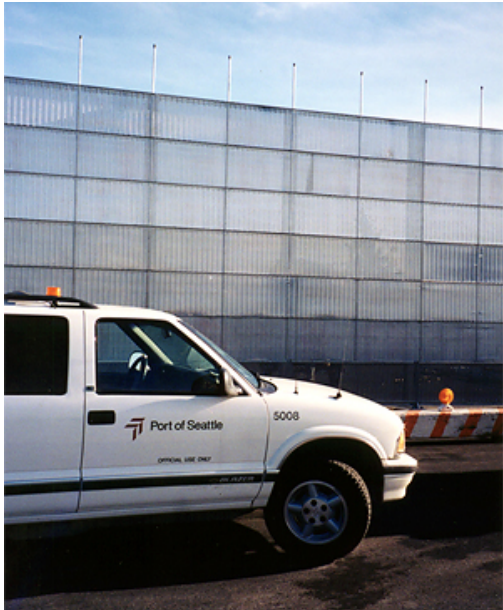
14-foot-high vertical fencing diffuses jet-blast from large aircraft while providing maximum perimeter protection.
