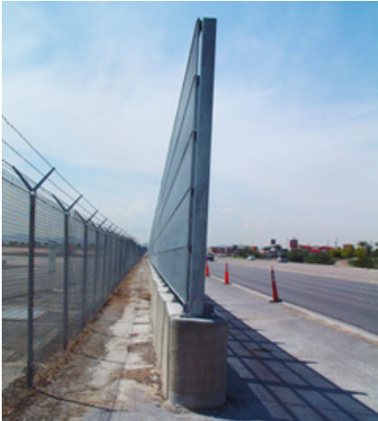
A narrow footprint (less than 24") allows placement in close proximity to other structures.
