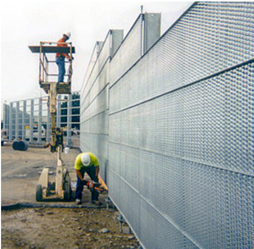
The Double-Reverse Corrugated (DRC) steel fabric controls heat and exhaust, moving it up and away from the fence.
