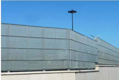
Angled posts allow the fence to follow tarmac irregularities, providing a significant cost savings over other systems, which must stop or overlap when faced with changing direction.
