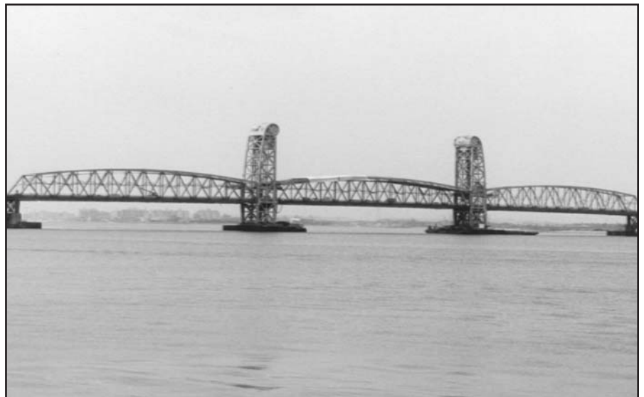
Marine Parkway Bridge
