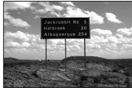
One of the 3 post signs in Arizona with Break-Safe® Couplings
