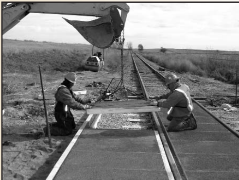
Crew lowers a precast polymer concrete panel into place
