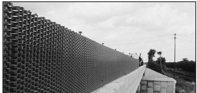
Clint Moore Bridge, Palm Beach County, Florida
