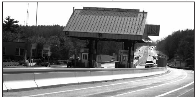
The yellow visi-stripe cautions drivers to slow near the toll plaza
