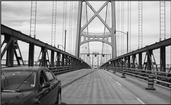
Bridge left lanes with T-48 overlay, right lane awaits coating.
