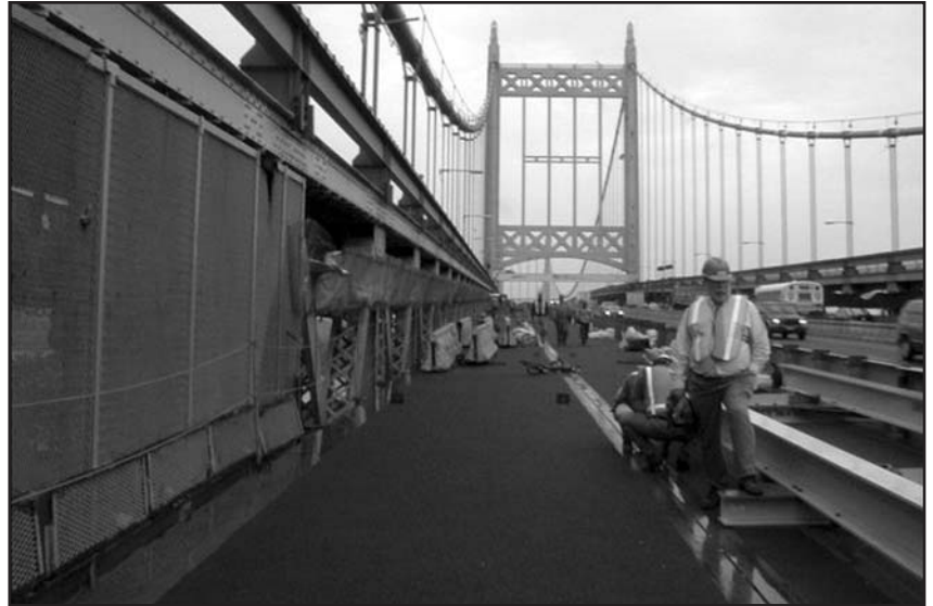
Workers placing T-48 overlay on the bridge deck
