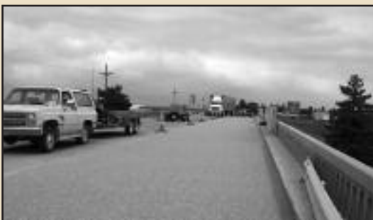
6,200 square feet of T-48 was applied in about 2.5 hours
