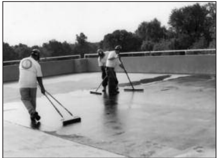
16,000 square feet of Sealate® was applied in just 3.5 hours
